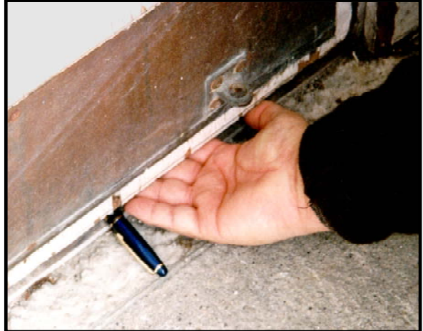
Figure 10: This gap at the bottom of the door is large enough to allow rat and mouse access to the building. Installation of a door sweep would exclude rodents.
